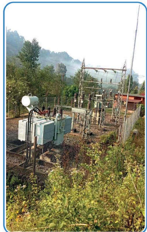
Tadi Khola HEP Tadi Switchyard
