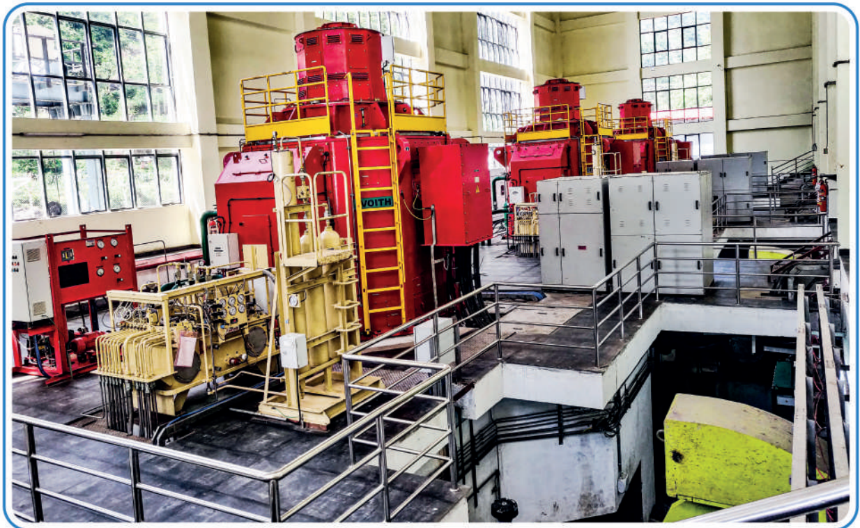
Mistri Khola HEP-Power House Generators
