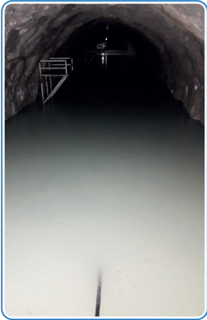
Mistri Khola HEP - Desander Basin during operation
