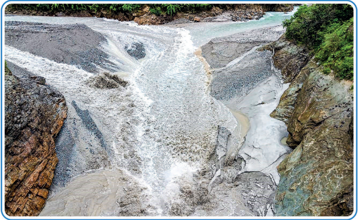
Mistri Khola HEP-Reservoir flushing
