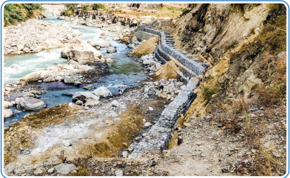
River Training for TL Tower Protection along Kaligandaki river
