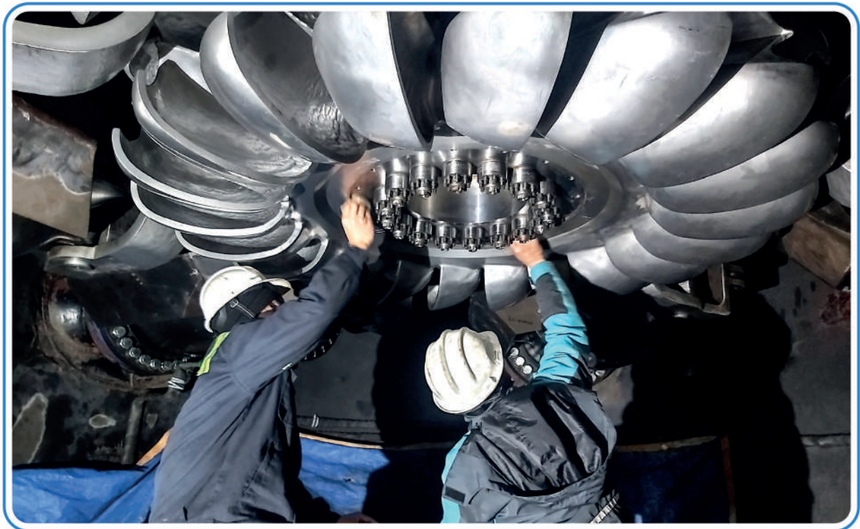
Mistri Khola HEP - Replacement of New Runner
