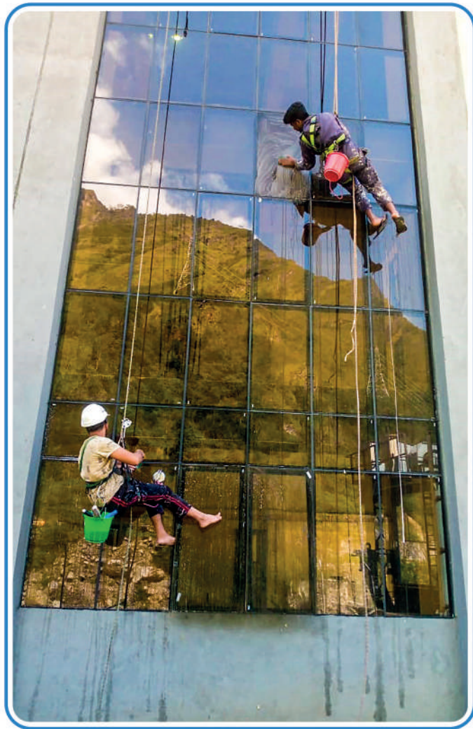
Mistri Khola HEP - Power House Cleaning work
