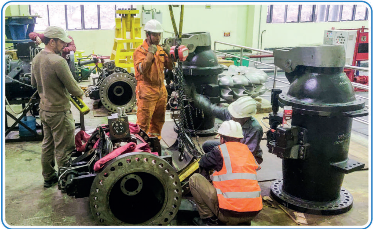
Mistri Khola HEP-Nozzle Servomotor Maintenance
