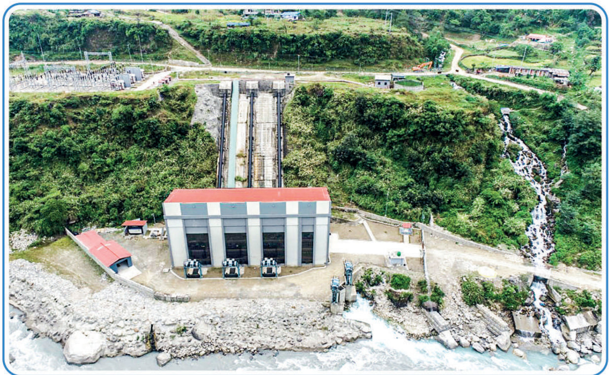
Tailrace Tapping for Mistri2 Diversion
