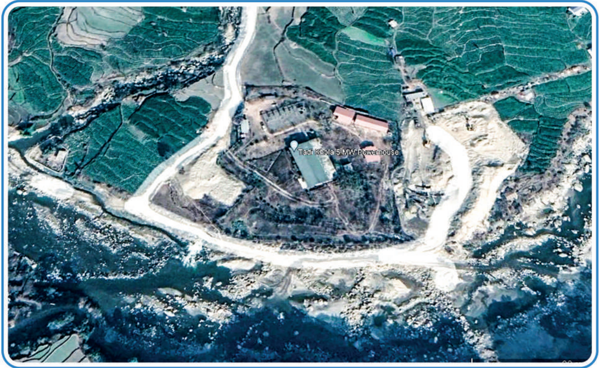
Aerial view of Tadi Khola Powerhouse
